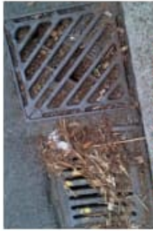
DRAINAGE SYSTEM MAINTENANCE
